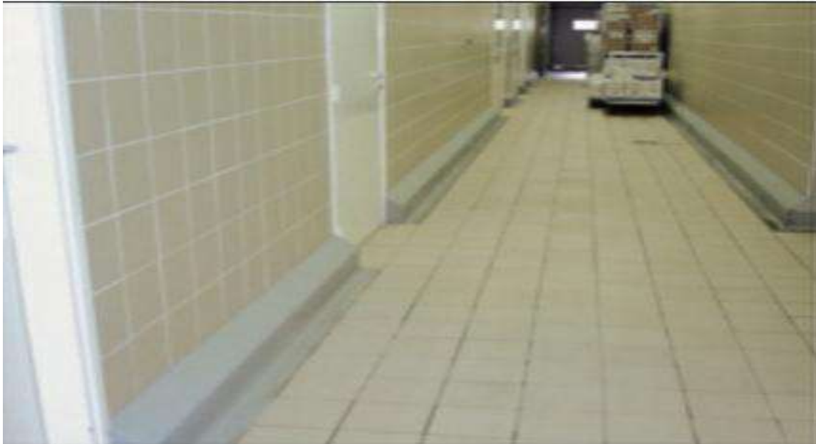
Figure 6: Banquette de protection murale
