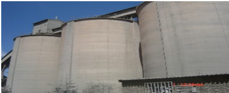
figure ( 7): silo de stockage ciment.
