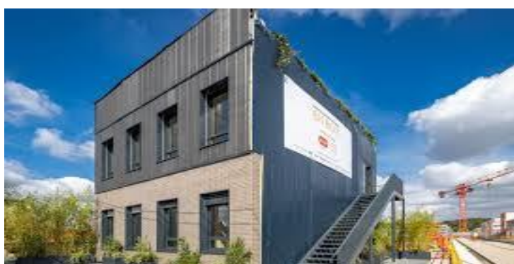
Figure 6. Bouygues construction cleanup
