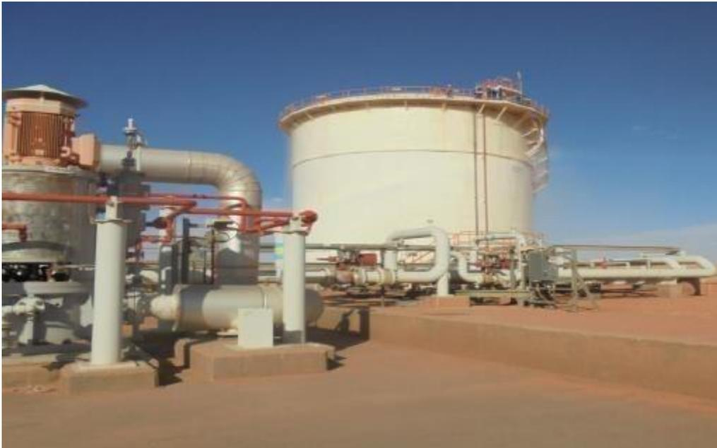
*Figure 23 : Stockage de condensat on-spec.*
