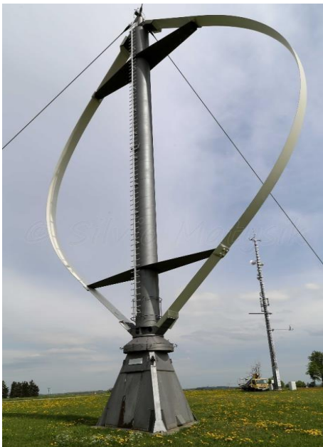
Figure II.3 : Eolienne de Darrieus
