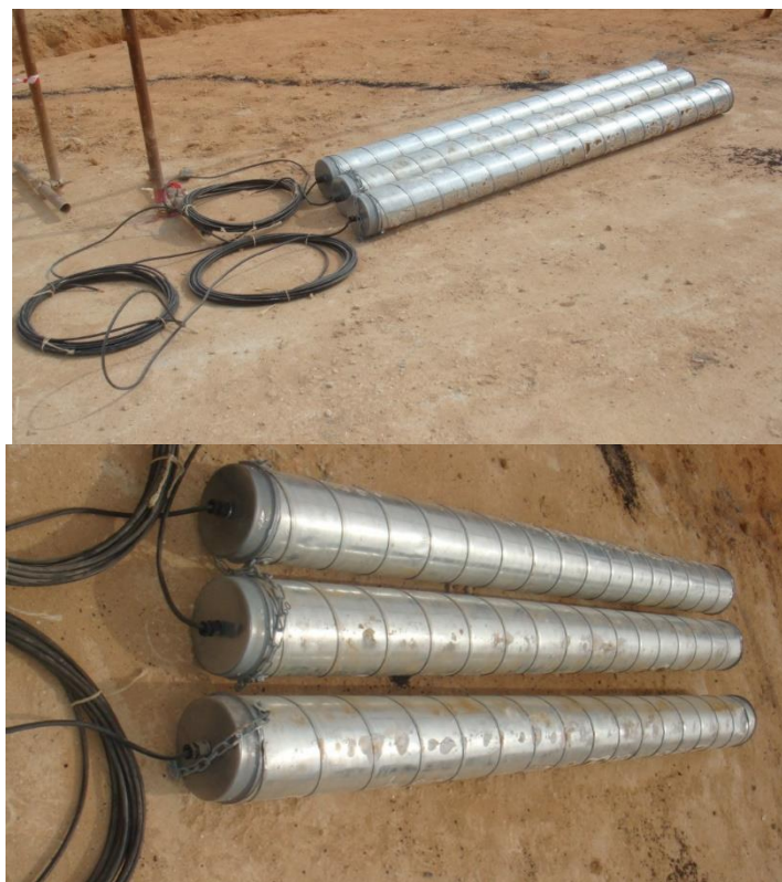
Figure III.1 : Anodes de types ferro-silicium.
