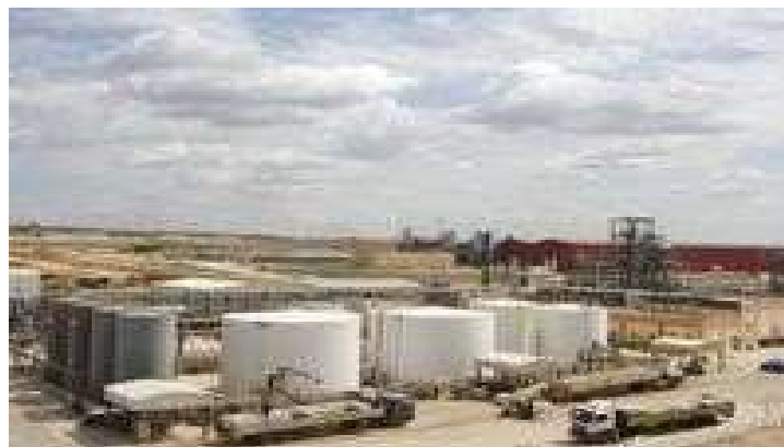
Figure IV.8 Usine de chlore
