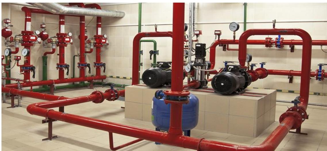
Figure 2-22: Installation sprinkleur [24]
