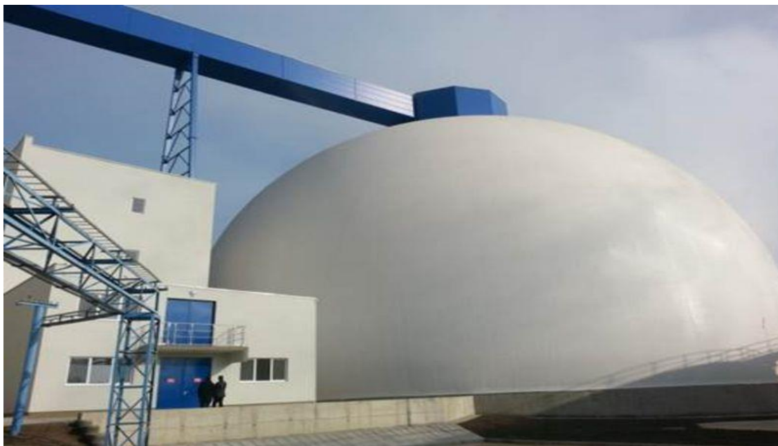
Figure 16 - Silo de stockage de type "dôme"
