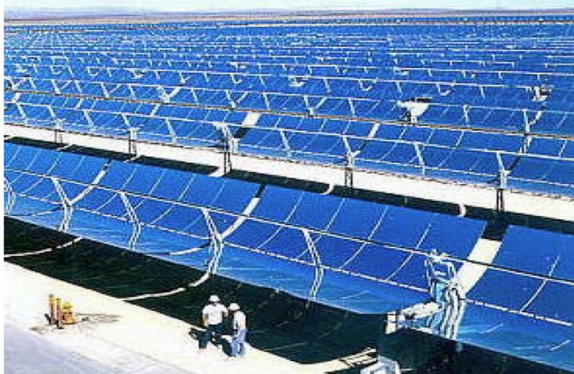
Figure 1-2 :The Solar Energy Generating Systems (SEGS) solar trough farm at Kramer Junction, California.
