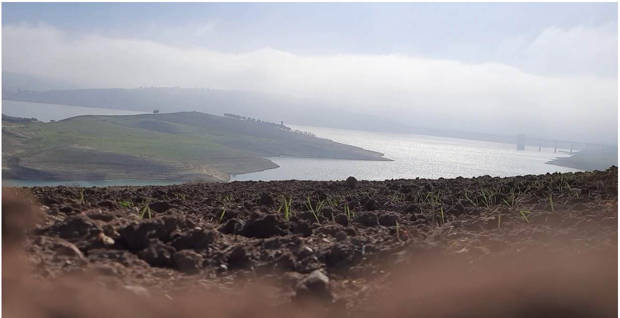
Fig.04 : Barrage de SIDI ABDELLI (B. Bouzid, photographe, 2015).
