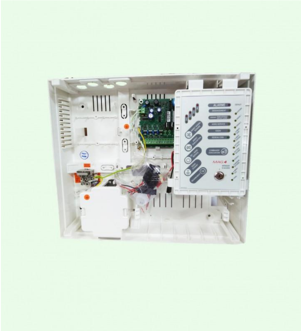
Figure III.1 : Centrale MAG4 (vue interieure)
