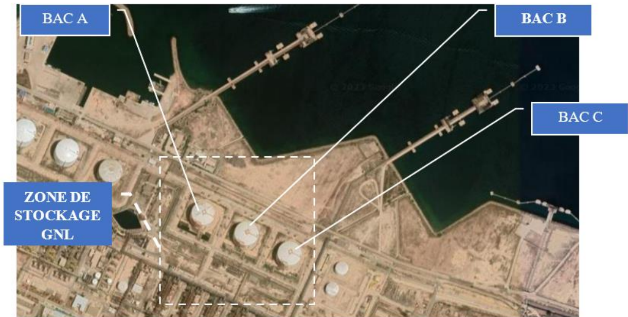
Figure IV. 8: Bacs de stockage GNL / GNL2Z
