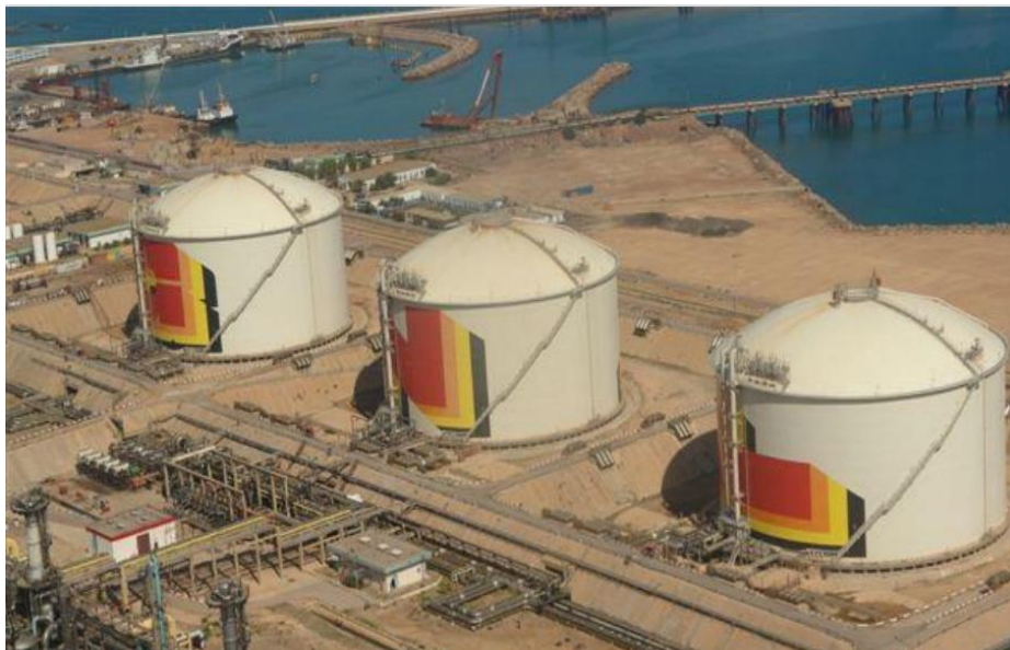
Figure III. 7: bacs de stockage de GNL /GNL2Z
