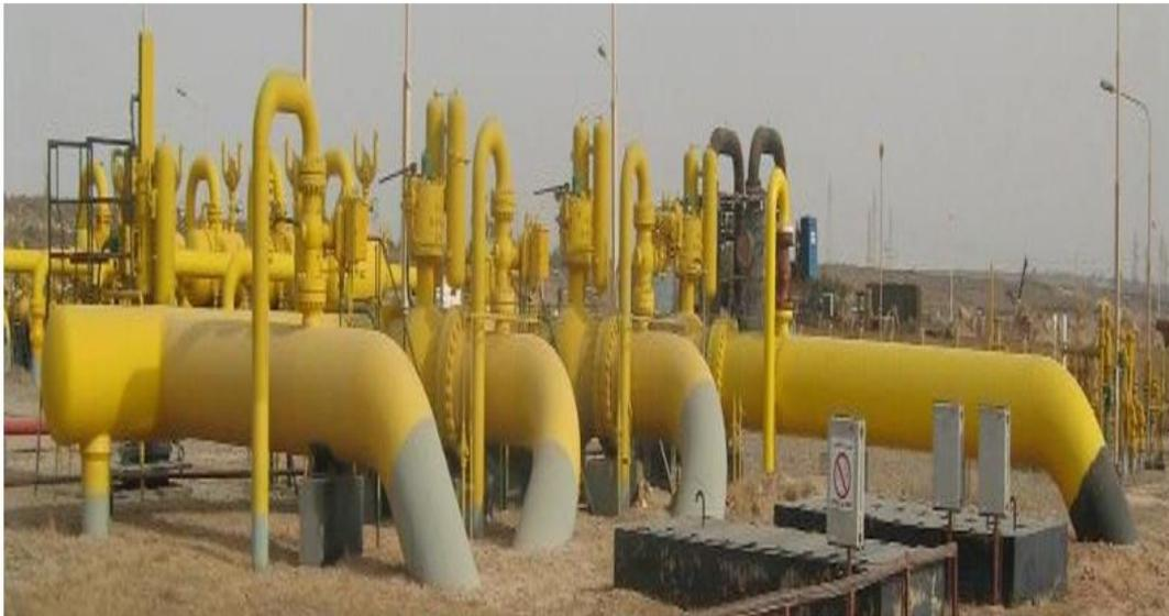
**Figure 19.** *Manifold D'interconnexion.* [F21]
