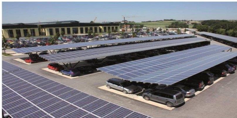
Figure I.6 Ombrières photovoltaïques
