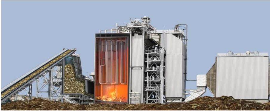
Figure 1.10 : La centrale Biomasse [34]
