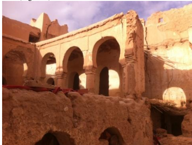
Fig4 example of a deteriorated house of Moussani
