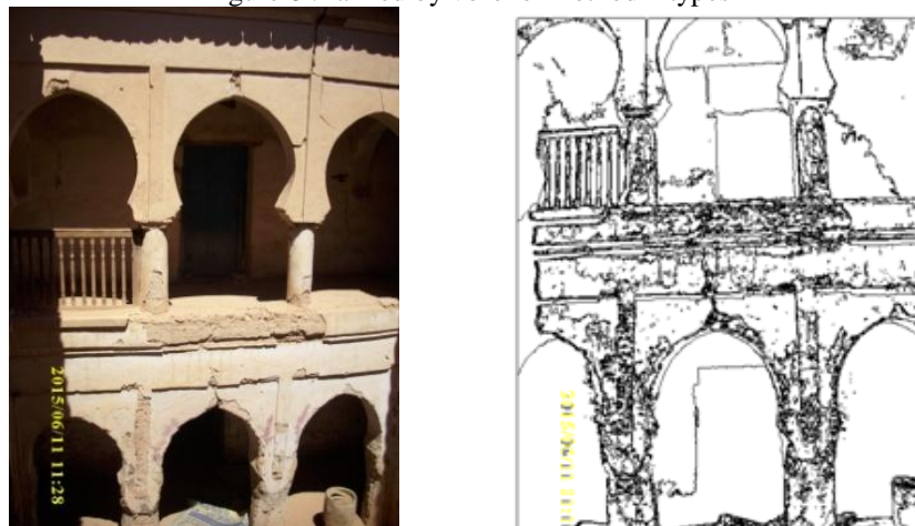
Figure 9 : interior facade of the Ksar with the vectorization of the image
