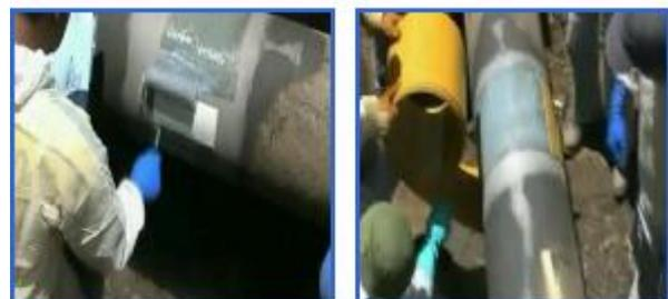
**Figure II. 6** : installation de Clock Spring [22]
