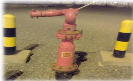
Figure IV.5 : Lance monitors (Rekkab M,2023)
