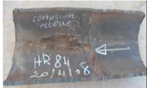
Figure 20 : Percement de manchette de transport
