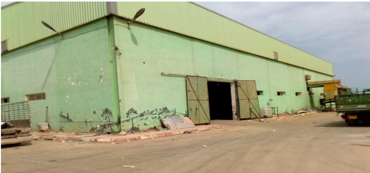
Figure II.10: hangar de tri.
