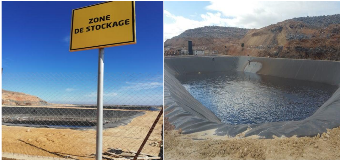
Figure II.12 :bassin de lixiviat.
