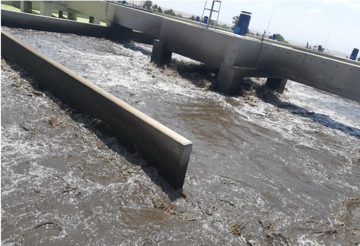
FIGURE III.9 BASSIN D'AERATION
