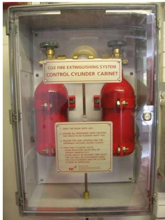
*Figure 68 CO2 System Release Control Cabinet*
