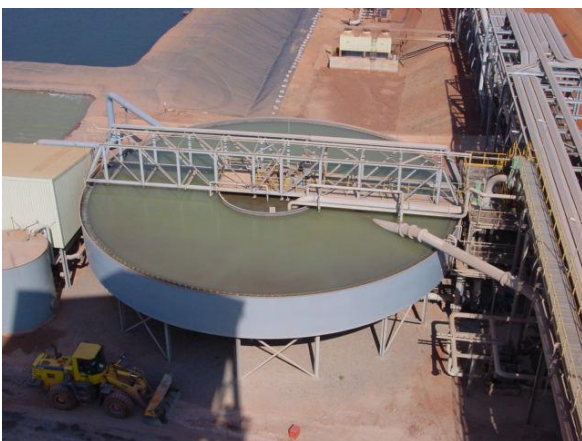
Figure33: Epaisseur ou thickener (Source: processing department, TMLSA)
