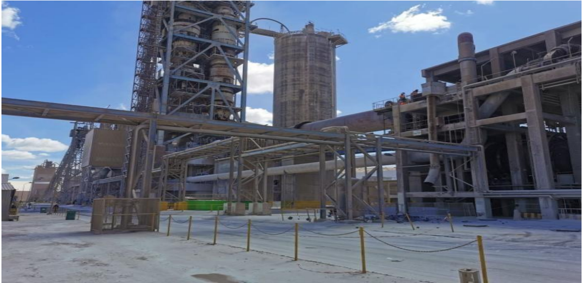
Figure 14: Exchanger a cyclone
