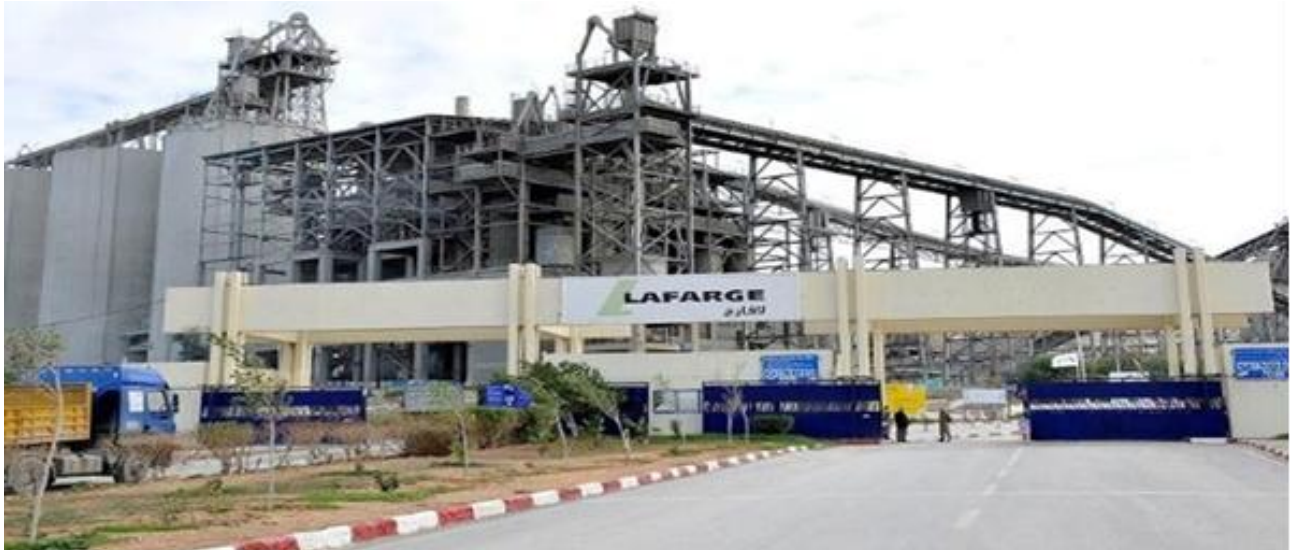
Figure 10: Cimenterie LAFARGE Ciment Oggaz.
