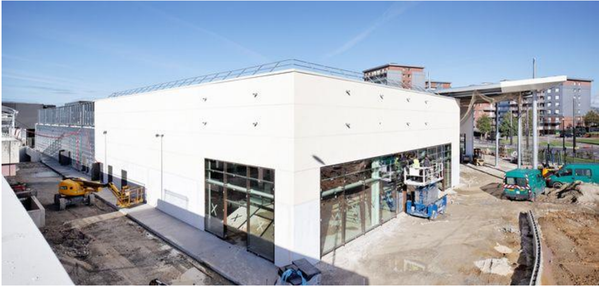
Figure 3. Chantier d'un centre commercial [21]
