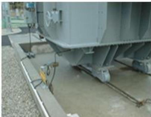
Figure III- 18 Protection masse cuve.
