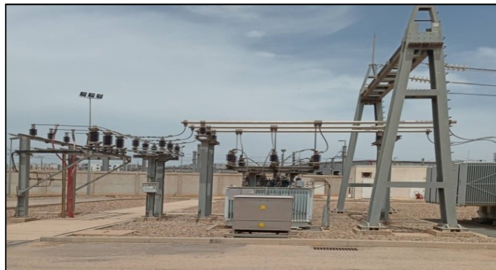
Figure II.2.1 - Point Neutre Artificiel
