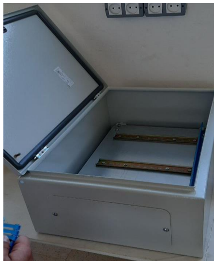
Figure 3.8 : Fixation de rails [19]
