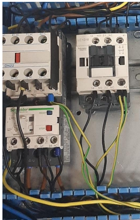
Figure 3.19 : Raccordement de relais thermique
