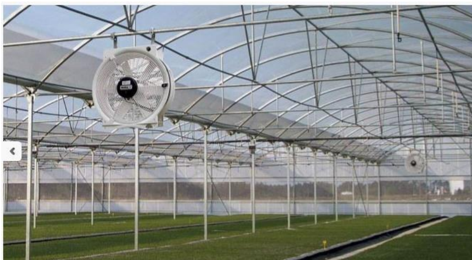
Figure I. 12: La ventilation horizontale
