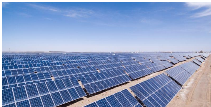
Figure 2.3: El Kheneg Solar Plant (Laghouat).
