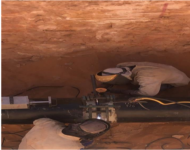
Figure 2 .6 Application du soudage SWAM
