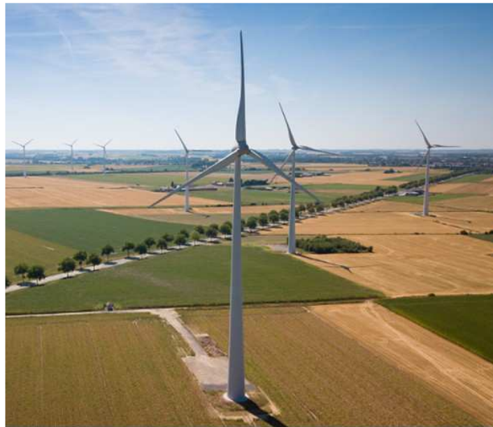
Figure I.4: Onshore wind turbine installation. [23]
