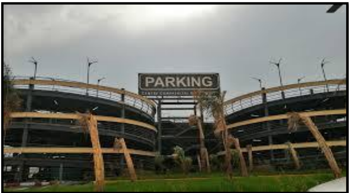
Figure 29: Parking du centre commercial ES-SENIA source (Google photo)
