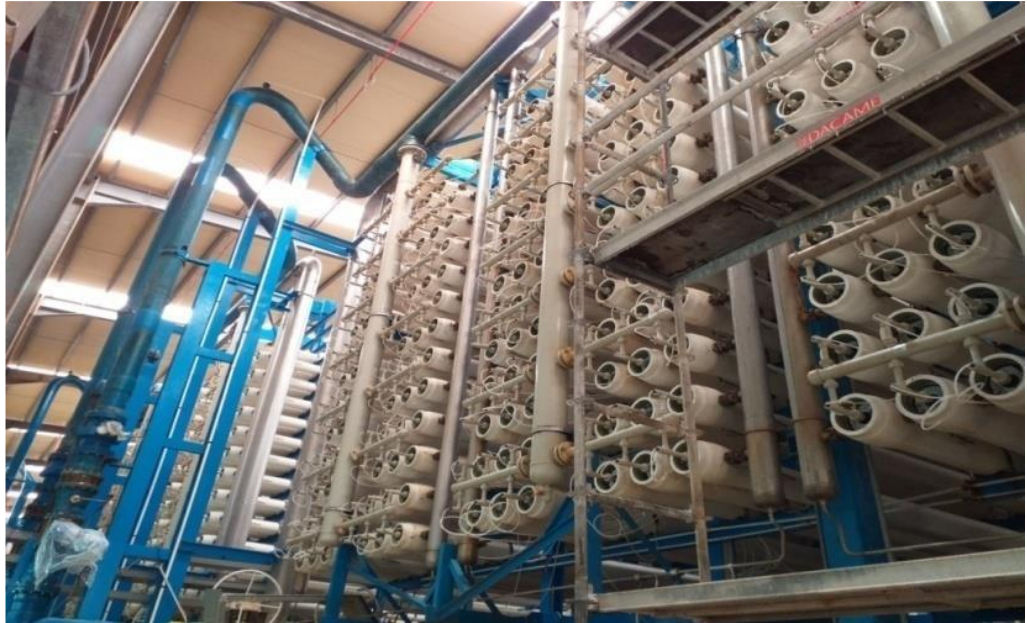
Figure II. 10: Les tubes de pression
