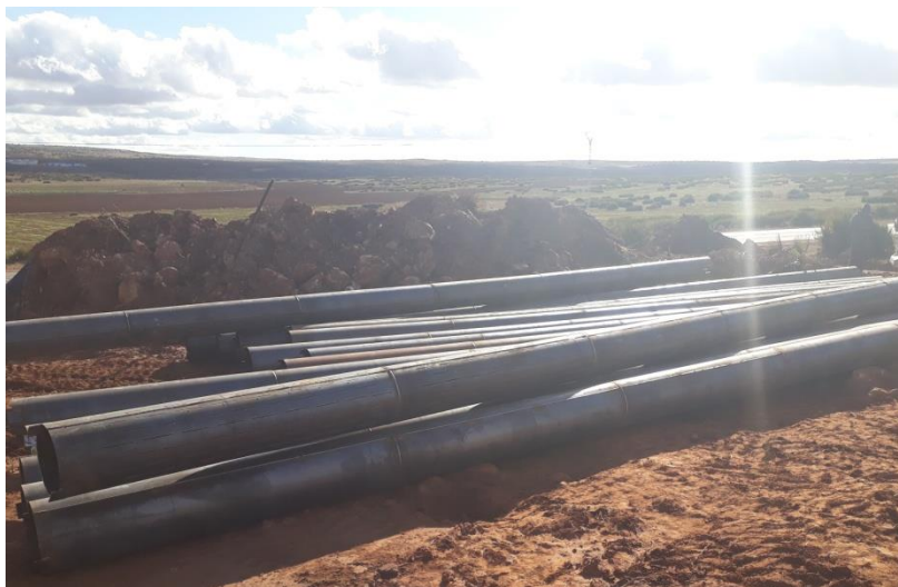
Figure 24 : Tubes pleins 13 3/8 (sur chantier)
