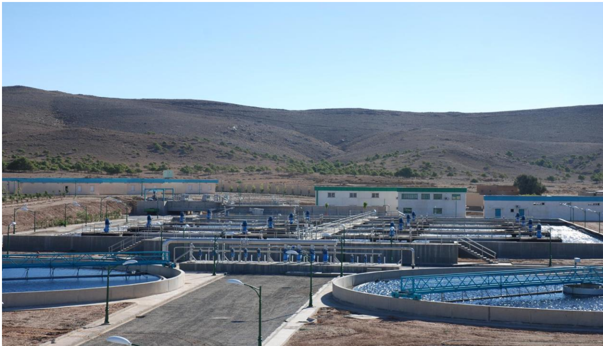
Figure 20: station d'épuration d'El Bayadh
