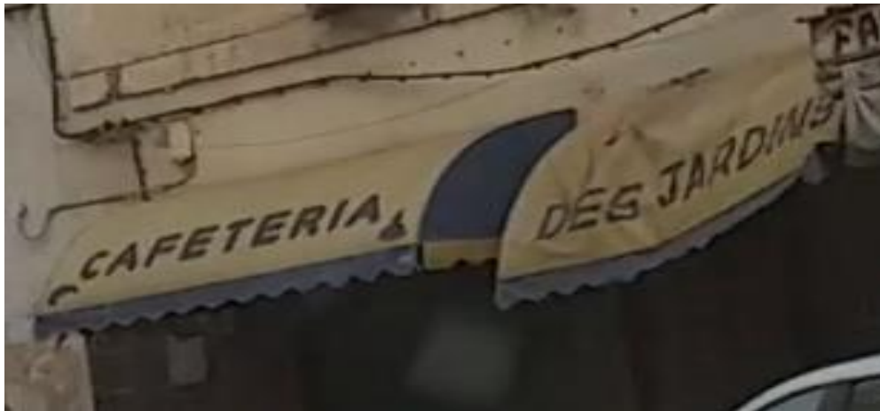
Pic 4.47: Cafeteria's shop roof (Sidi El Houari).
