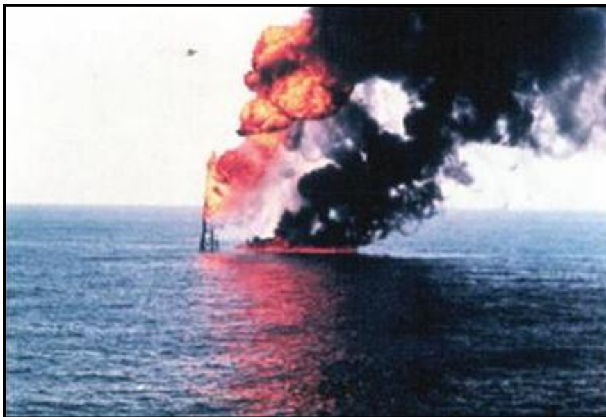
Figure 5.2.c Flaming liquid engulfs flare stack.
