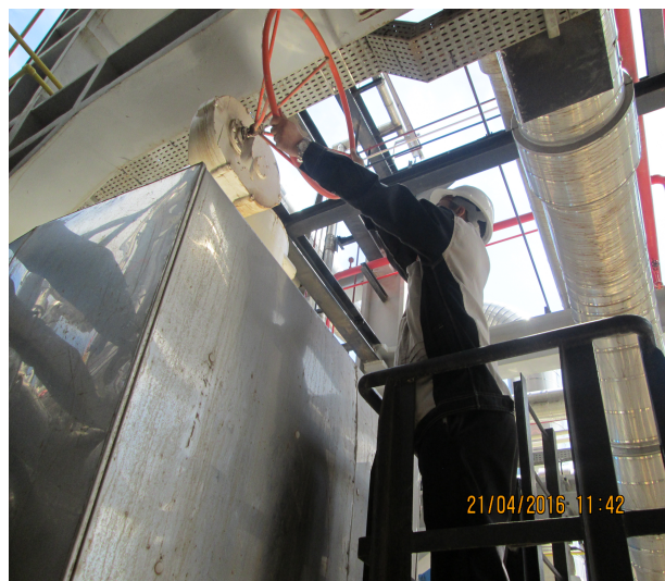
Figure 25.30 vanne inaccessible
