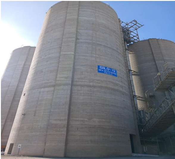
Figure 1.20: Silos ciment (ligne 3).
