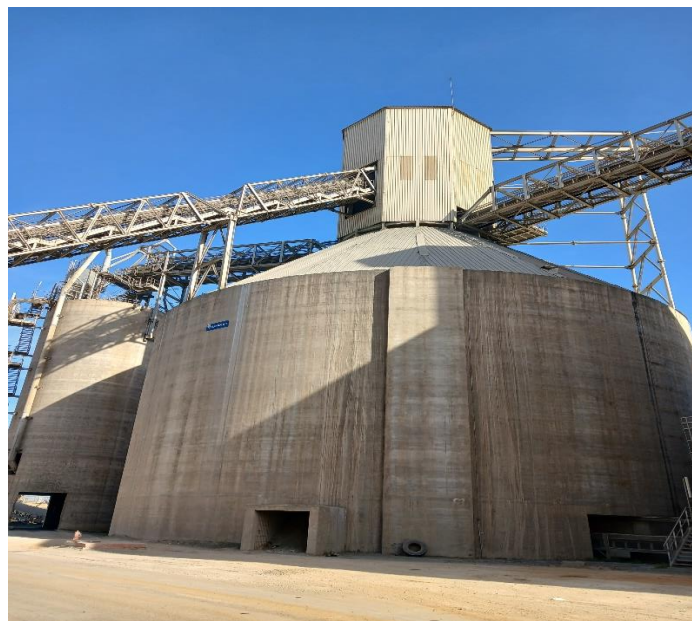
Figure 1.18: Silos clinker (ligne3).
