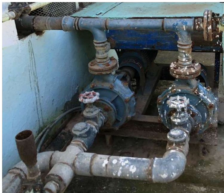
Figure II.15 : Pompes d'arrosage.
