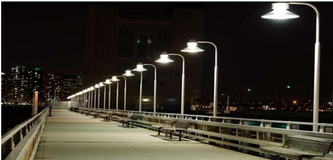
Figure 1.1: Example of street lighting
