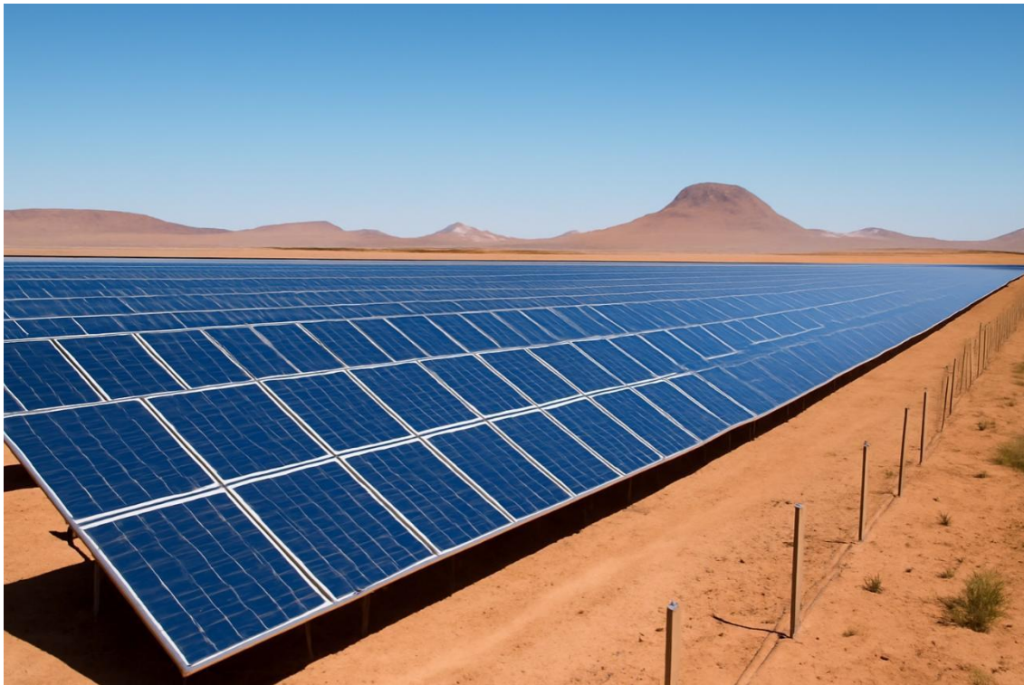
Figure 1 centrale photovoltaïque algérie hassi r'mel
