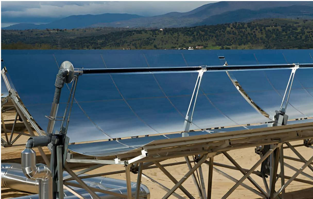
Figure 2.9 Parabolic trough collector [44]
