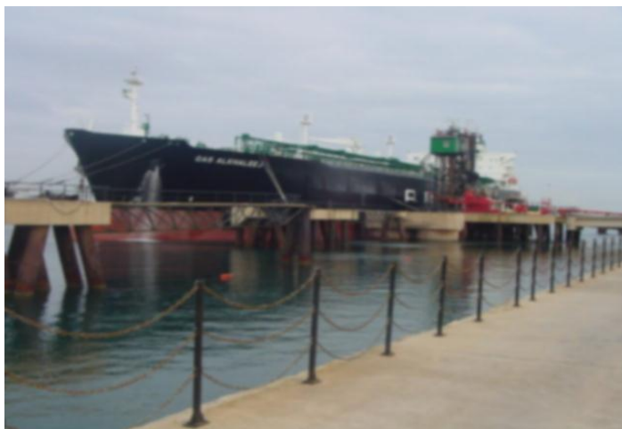
Figure 1.7- Quais de chargement [4].
