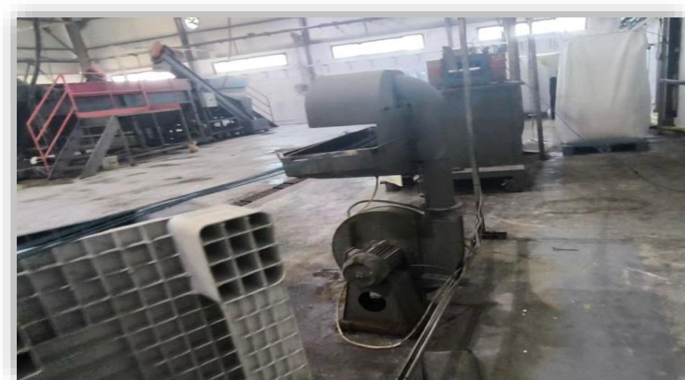
Figure II.12 : Operation de suchage
