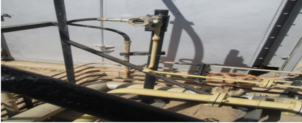
Figure II. 15: transmetteur de gaz PTH
