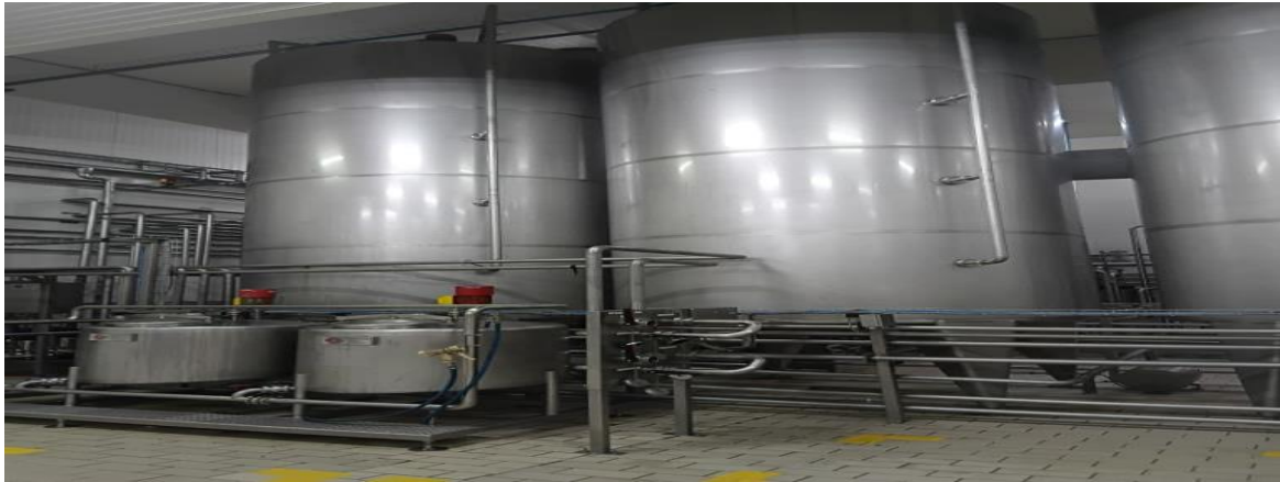
Figure 2-2:Cuves de fermentation
