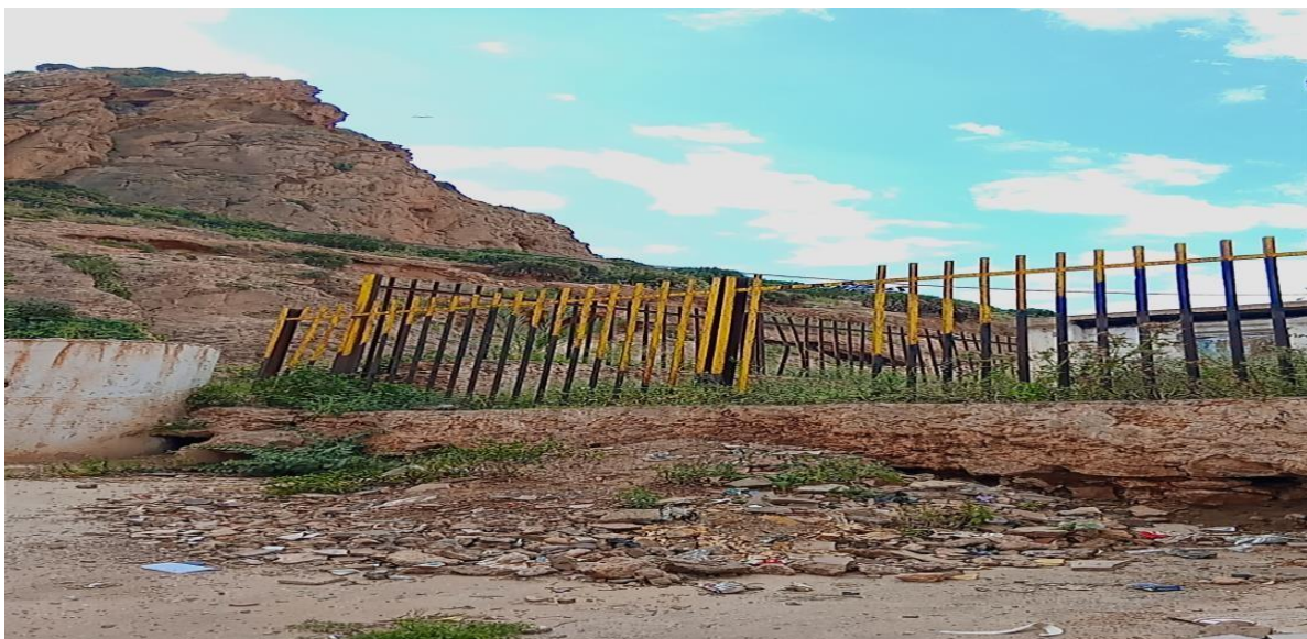
Figure 37 : point du captage la source El-Ançor.
